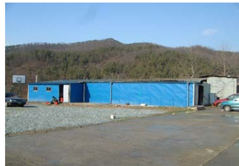
Fig 2. Photograph of the test facility
