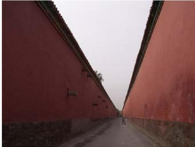
**Figure 7:** Fire separation and fire road in the Peking Imperial Palace.
